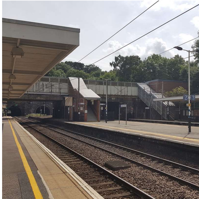
Figure 41: Hadley Wood railway station (source: Troy Planning)
