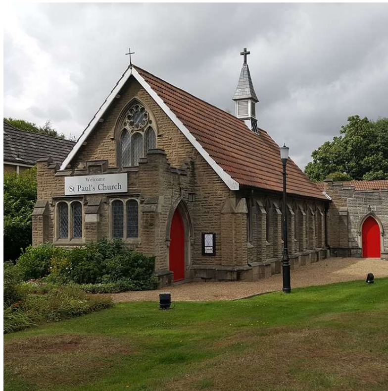
Figure 38: St Paul's Church, Hadley Wood (source: Troy Planning)
