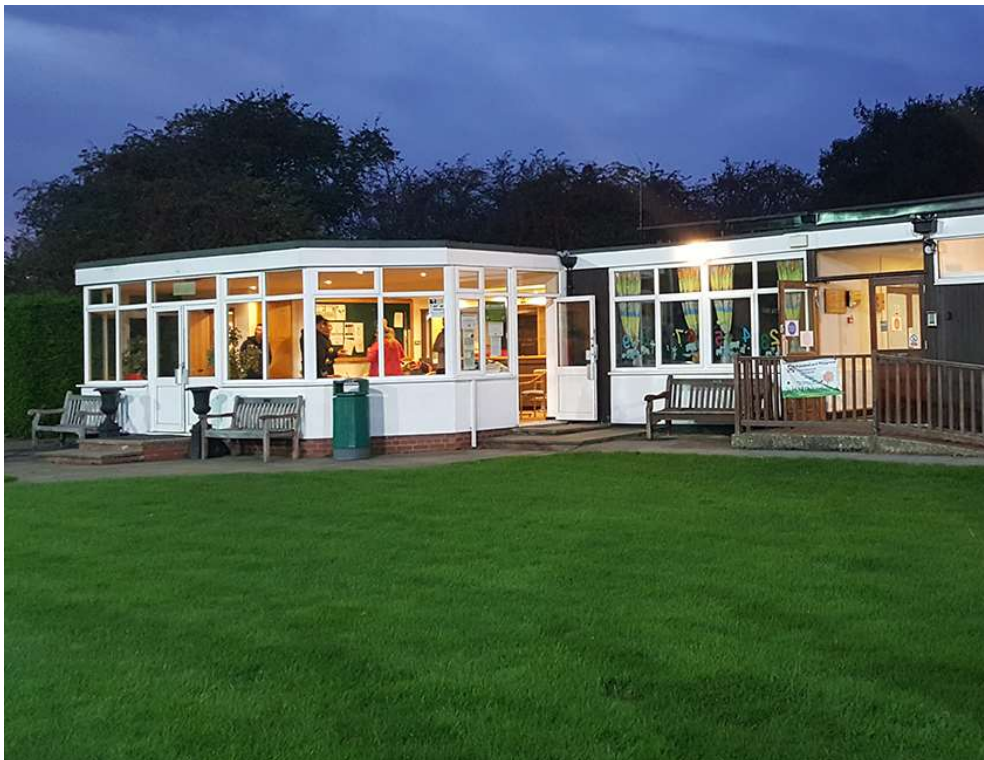
Figure 39: Hadley Wood Association Centre (source: Troy Planning)
